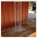
The average size of the concrete base will be 2'x2' but may vary slightly depending on the height of the tower. Once the base is built, the concrete will need to fully cure before we can come back and stand your tower.
